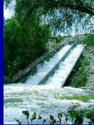
Dos Rios recycled water outfall
